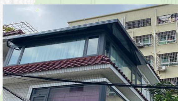
Insulated panel sun room
